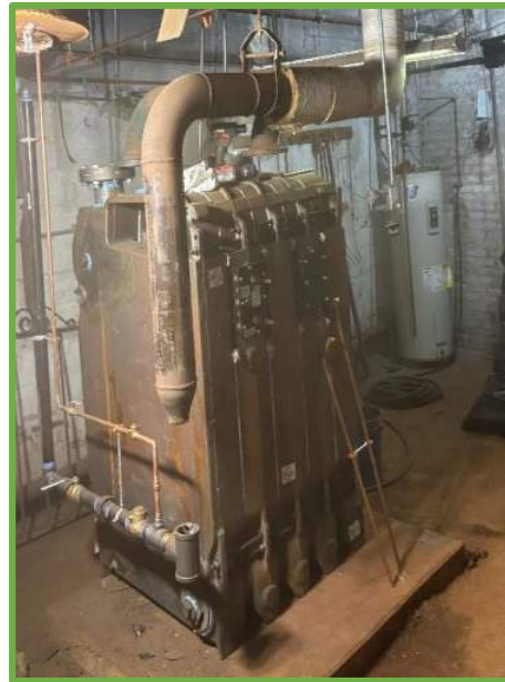
Installation of new boiler
