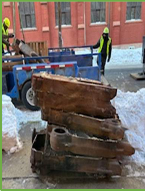
Removal of old boiler
